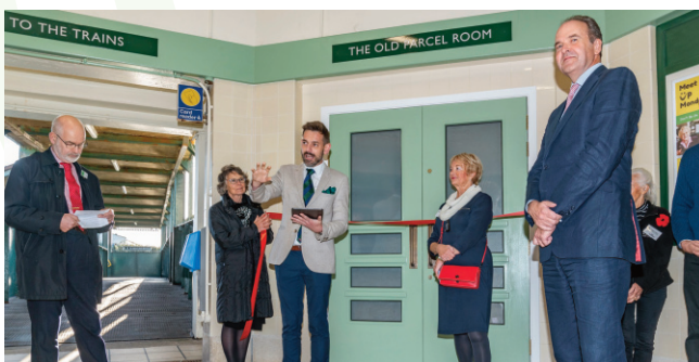
The Friends of Bishopstone Station have led on the renovation of the station's 1930s former parcels office, revamping the space as a community hub.
