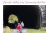
Amber Cutting Tunnel, Mansel Trail David Walker
